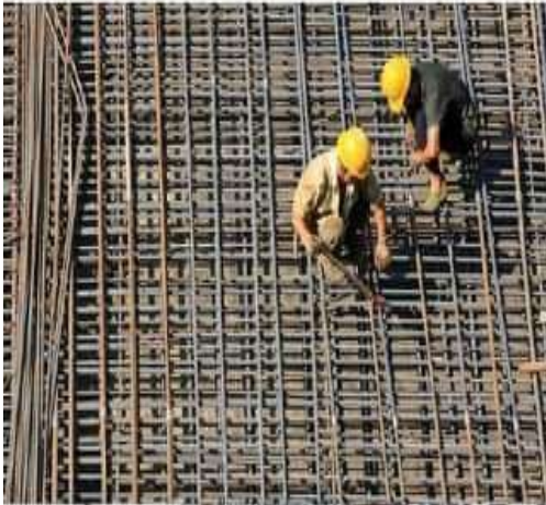
Steel reinforcement Work
