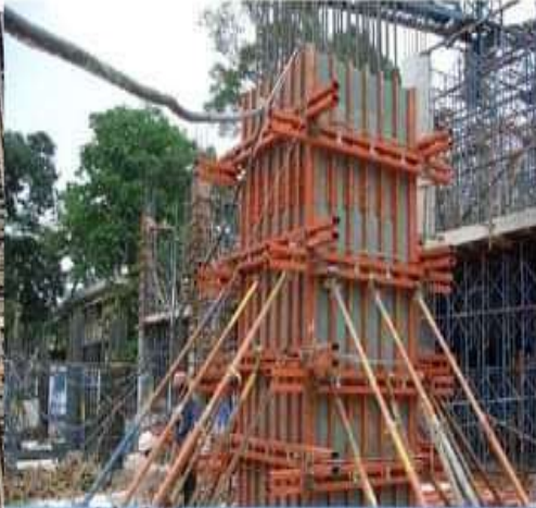
Formwork (Shuttering) Work
