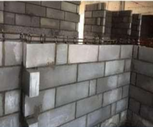
AAC Block & Bricks Masonry Work
