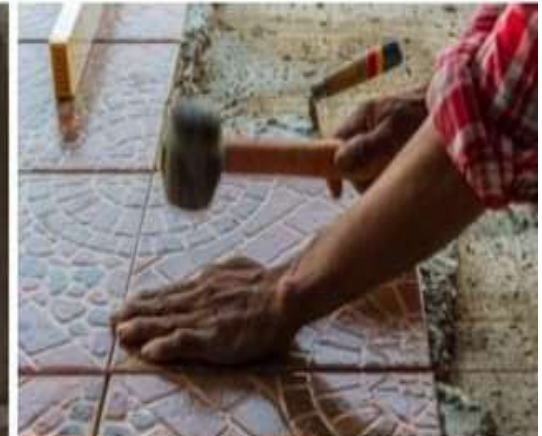
Flooring (Tiles) Works
