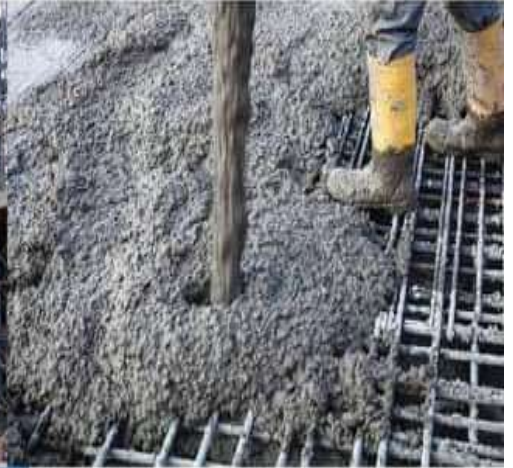
Pouring Concrete Work
